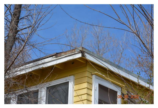
Figure 7. Deteriorated fascia board that provides an entry for wind-blown embers can result in an ignition on the interior of the structure.
