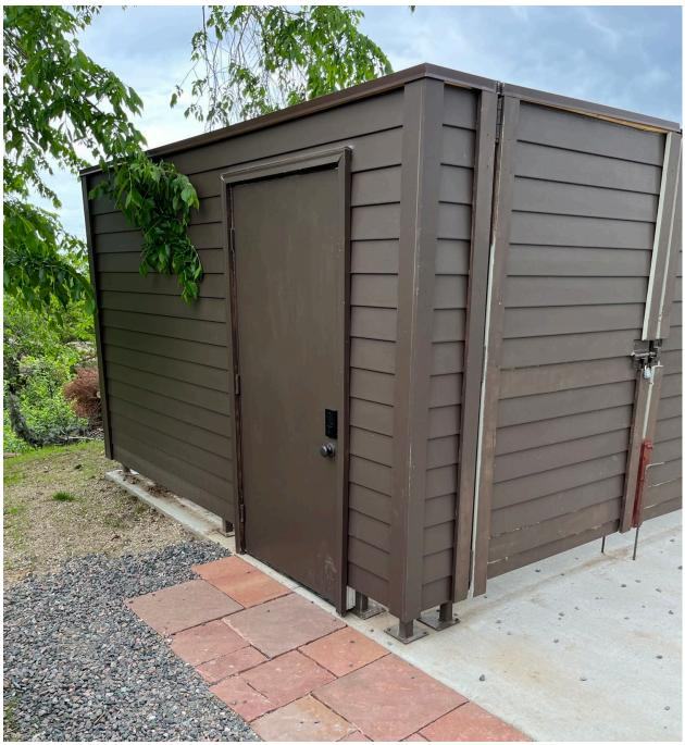
Figure 46: Fiber Cement Siding approved at new Chautauqua Trash Enclosure
