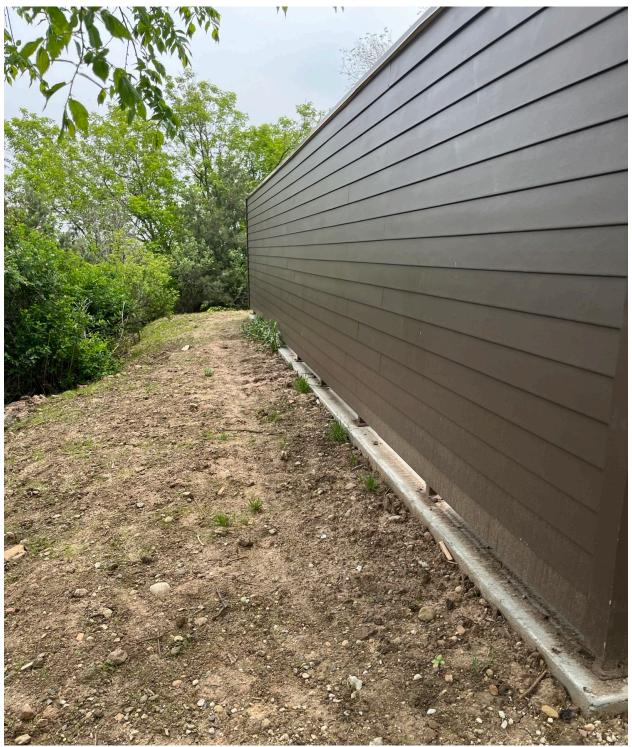
Figure 47: Chautauqua Trash Enclosure with Fiber Cement Siding
