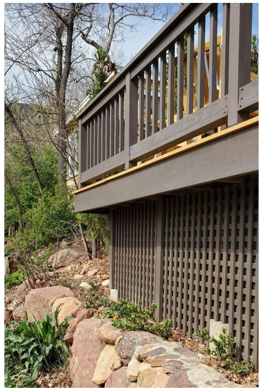
Figure 13. Mary H. Galey Cottage deck enclosure. The enclosure uses fire-retardanttreated wood and metal mesh to reduce combustibility and the likelihood of large embers causing ignition under the deck.
