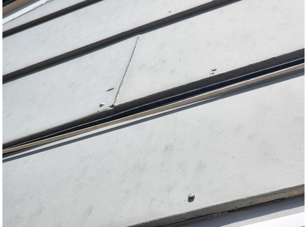
Figure 34: West Wall of 1957 Ranch in Colorado, Nails Visibly Working Their Way Out of Fiber Cement Siding (Lord, 2023)
