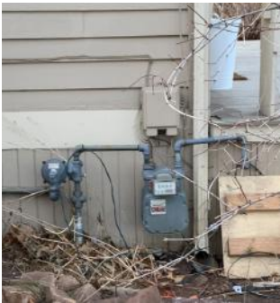
EXISTING GAS METER TO BE RELOCATED
