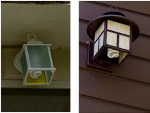
Various porch lights are installed throughout the dwellings and secondary buildings. Compact fluorescent and LED retrofit lamps are generally used.
