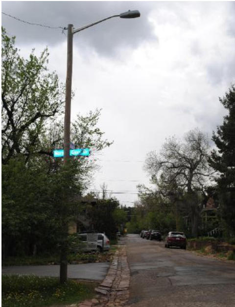
Figure G.3. The “Cobrahead” style street-light in this image is designed with a flat lens and does not emit light above a horizontal plane at the lens, it is FullCutoff. If it is mounted tilted up then that classification is compromised.
