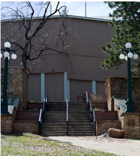
Gathering spaces and major building entrances are illuminated from acorn and multi-globe style luminaires on decorative poles. LED retrofit lamps are installed.
