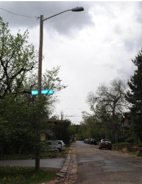
Cobra head luminaires with high pressure sodium lamps are mounted on wood poles for the majority of the street lighting.
